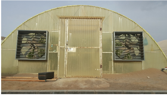
Figure 1. Quonset greenhouse with polyethylene covering and (a) fan-(b) pad evaporative cooling
