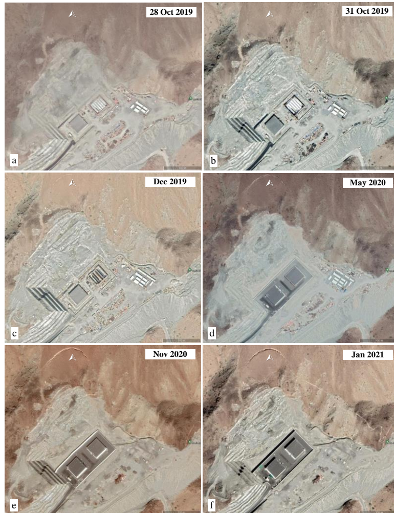
Figure 8. Satellite images (a-f) show that slope failure started between 28 and 31 October 2019 (a and b) as a result of major slope excavation and removal of the toe support in order to construct the tank.
