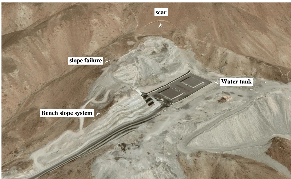
Figure 2. Landsat Google image (20 Mar 2021) showing the water tank and slope failure above it.
