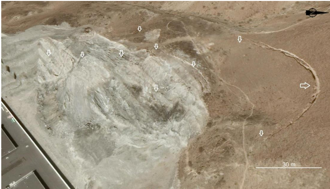
Figure 7. Collapse of benches initiating large fractures parallel to the main slide area.
