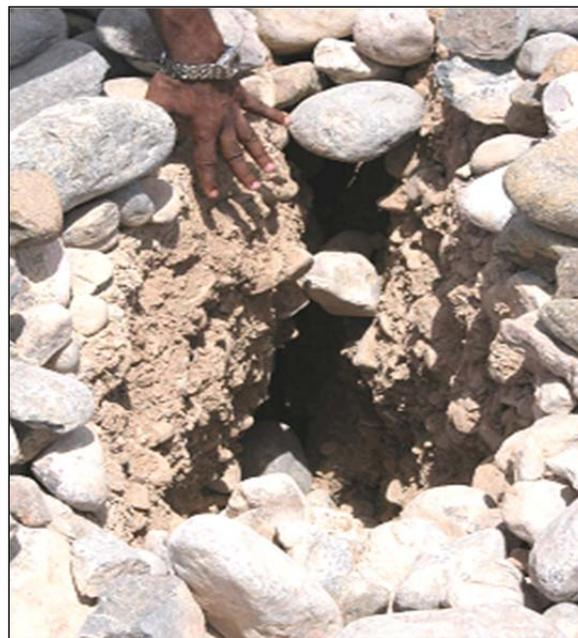
**Figure 5.** Crack in the crest of the dam at chainage 2+700.
