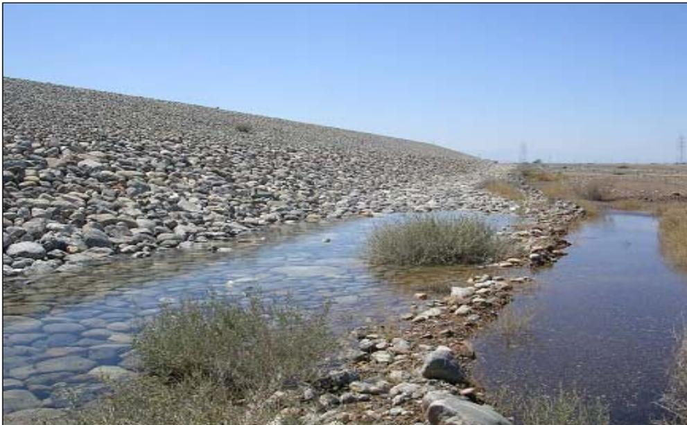
**Figure 3.** Seepage from the dam.
